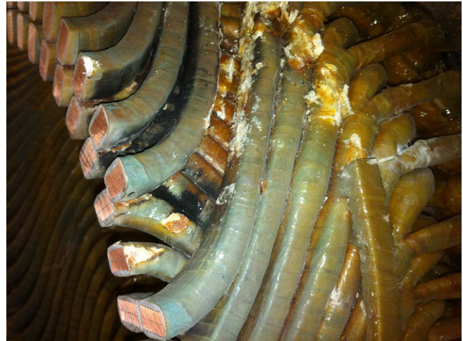
Figure 1. Aged Insulation System
