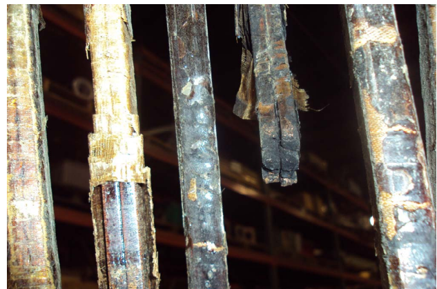
Figure 2. Failure Point and Surrounding Coils 2 nd Generator
